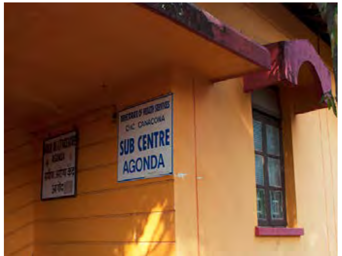
Medical dispensary, adjacent to the Panchayat's building, open two days a week
